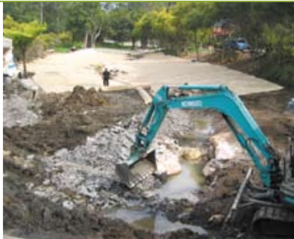
Tarban Creek during restoration
