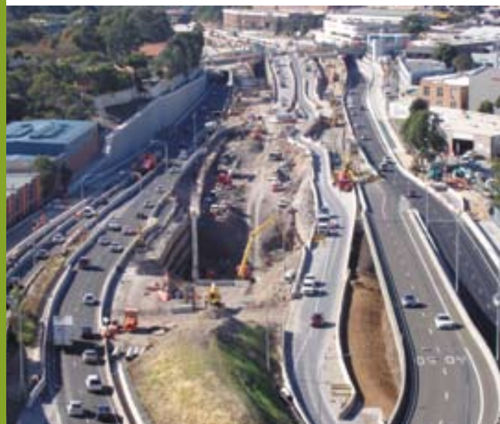
The Lane Cove Tunnel under construction
